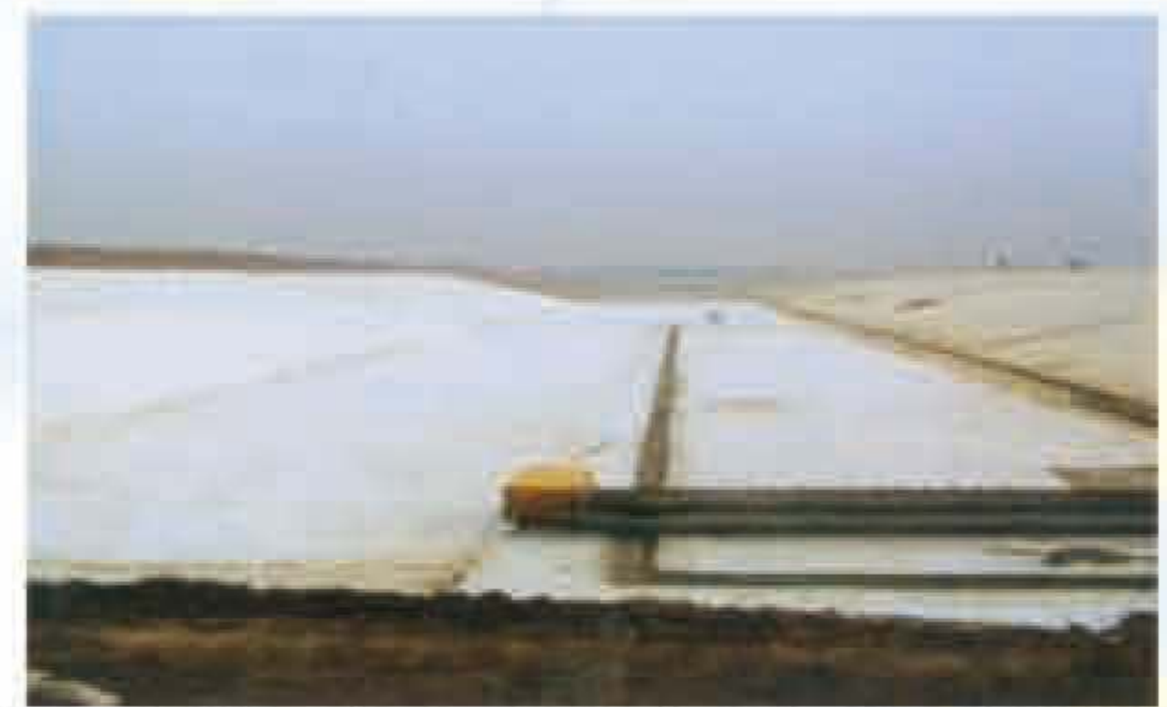
LDPE土工膜在南水北调工程中的应用 LDPE geomembrane in the South-North Water Transfer Project Application
