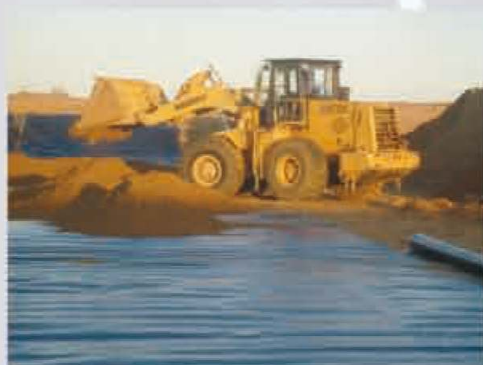
青海盐田防渗工程 Qinghai Salt Lake Anti-leakage Project
