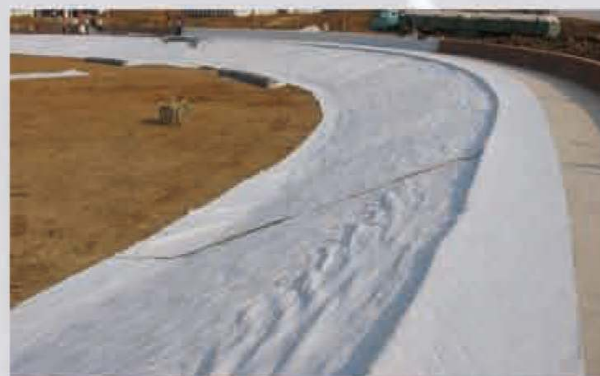
水库防渗 Reservoir Preventing Leakage
